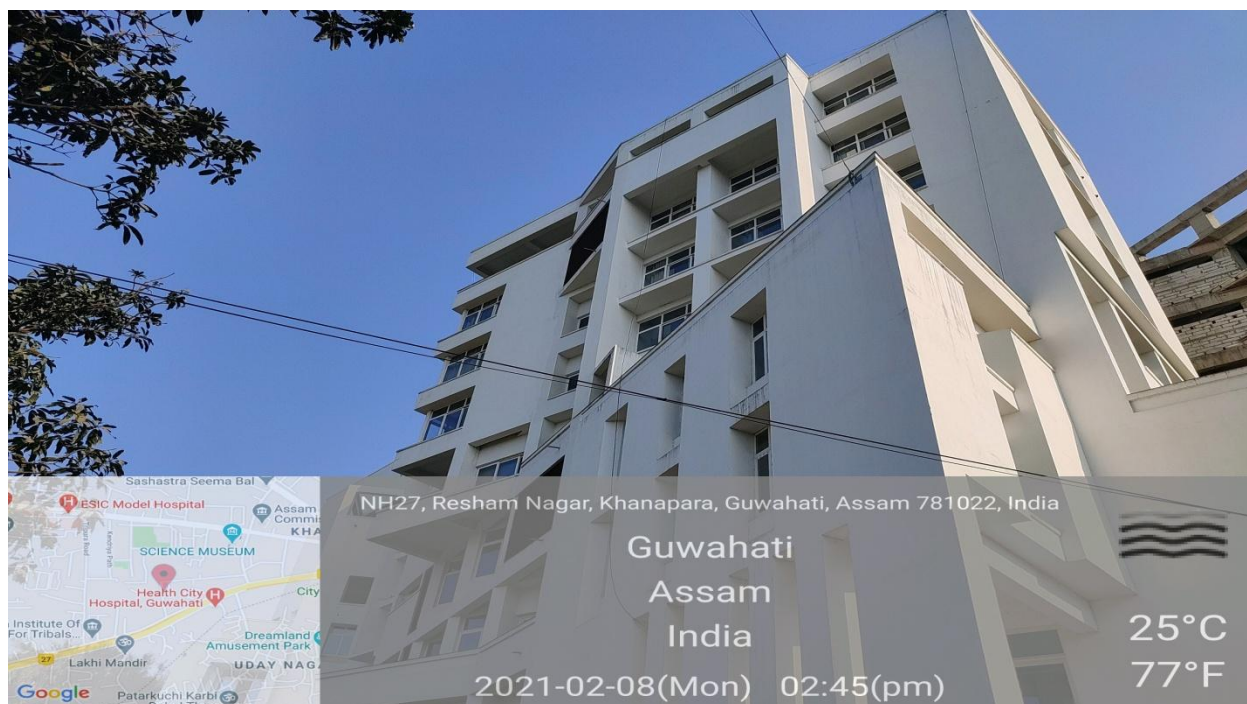
University City Campus Buildings, KKHSOU, Khanapara, Guwahati-22
