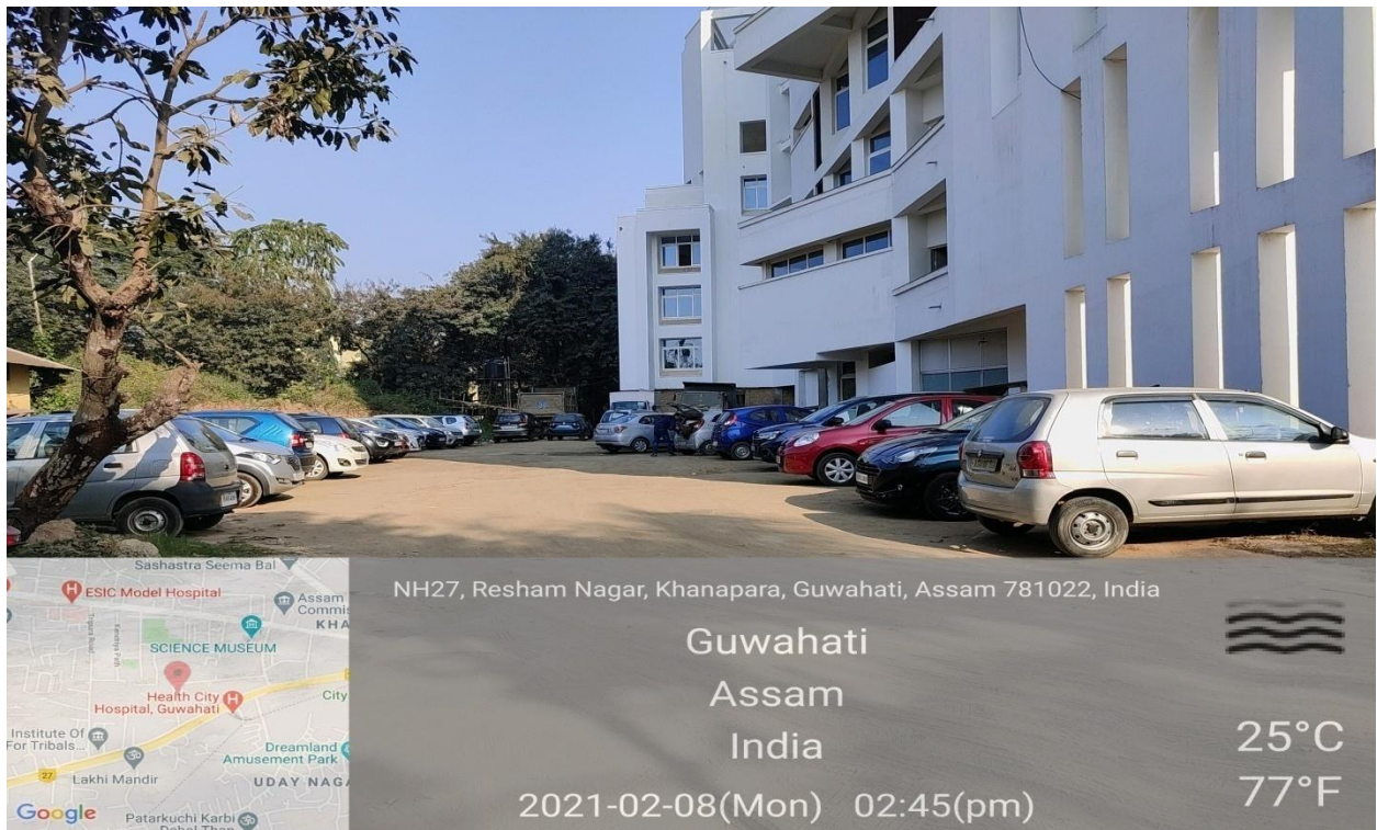
University City Campus Buildings, KKHSOU, Khanapara, Guwahati-22
